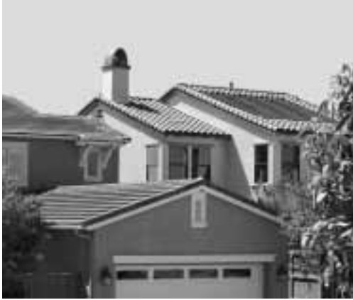
SunPower SunTile® Application on Three Rooftops
