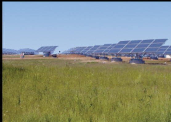
SunPower solar cells incorporated into Solon sun-tracking solar arrays, Germany
